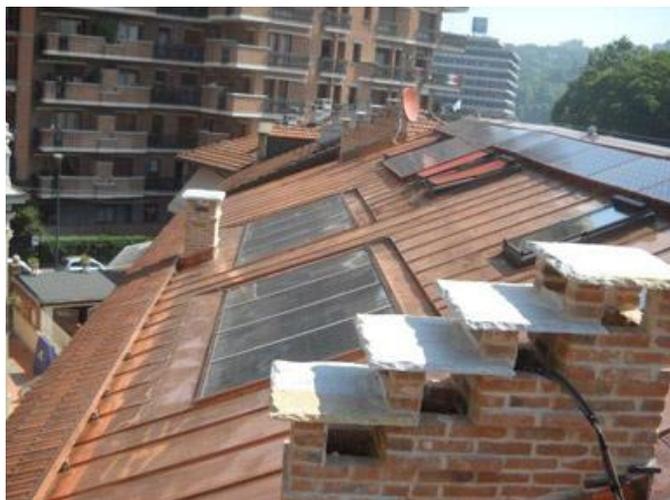
Figure 3 Roof view with the solar thermal and photovoltaic panels
